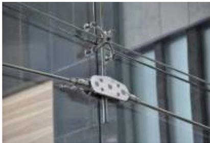
This decreases the amount of solid structural elements visible on the project, therefore increasing the transparency of the facade. The two main types in the industry are tension rod facades and cable net walls.
